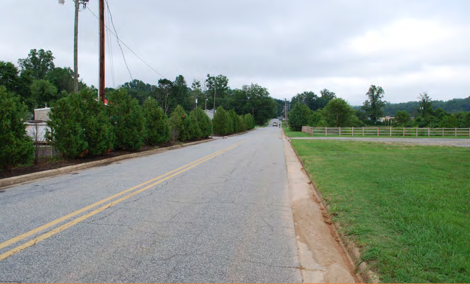
PENNTON AVENUE — EXISTING
